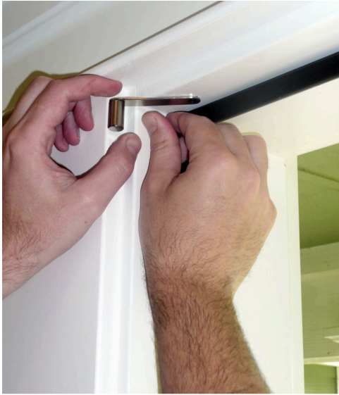
4. DEADBOLT SHOWN FULLY INSTALLED.
