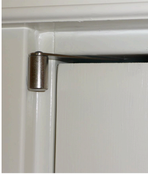
5. WITH DEADBOLT ROTATED TO "OPEN" POSITION (JAMB SIDE), CLOSE DOOR AND CHECK FIT OF DEADBOLT IN GAP BETWEEN DOOR AND JAMB. IF DEADBOLT RUBS, THE GAP IS TOO TIGHT AND WILL NEED TO BE ADJUSTED. (TIP: FOR WOOD DOORS, A BELT SANDER MAKES QUICK WORK OF THIS SIMPLE ADJUSTMENT).
